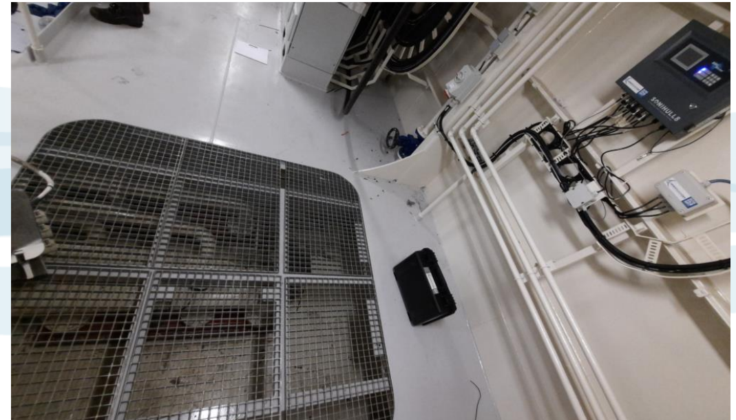
The installation as carried out on the TSHD. On the upper right, the control unit is visible, located above some of the box coolers.
