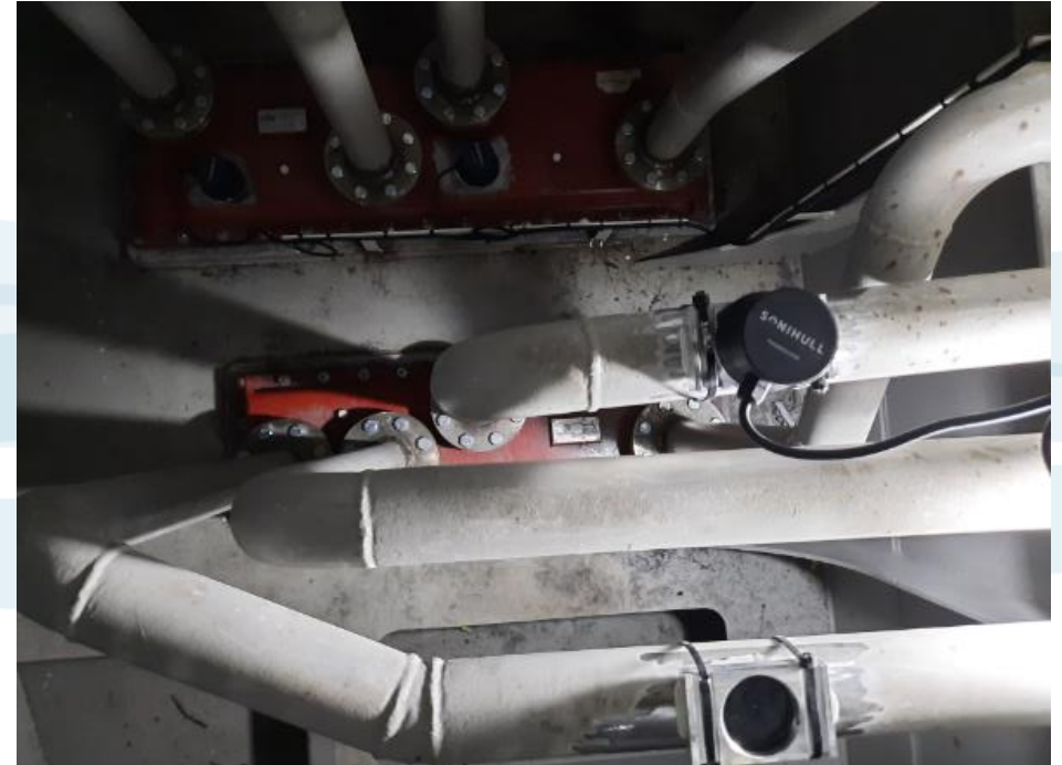
Two transducers are visible on the cooler cover. Two Pipe Adaptors can be seen in the picture, one of which has a transducer screwed into. To ensure optimal adhesion of the two component epoxy coating is removed. Following the curing of the epoxy, primer is applied to prevent corrosion around the mounting objects.
