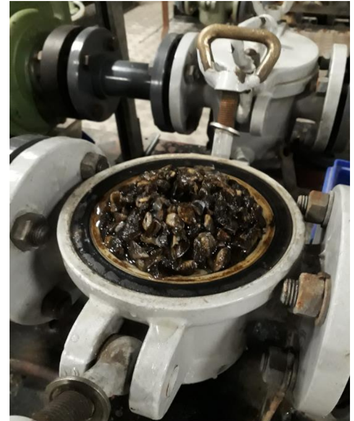
Clogged distribution filter
