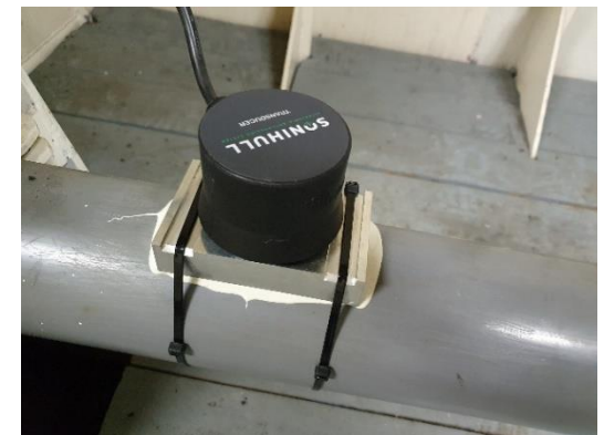
Transducer on a pipe with a pipe adaptor
