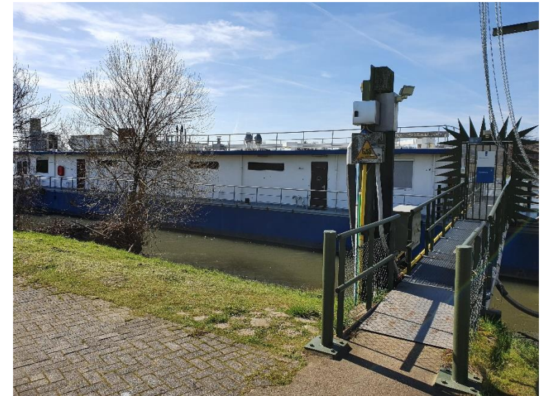
The RWS monitoring station in Eijsden
